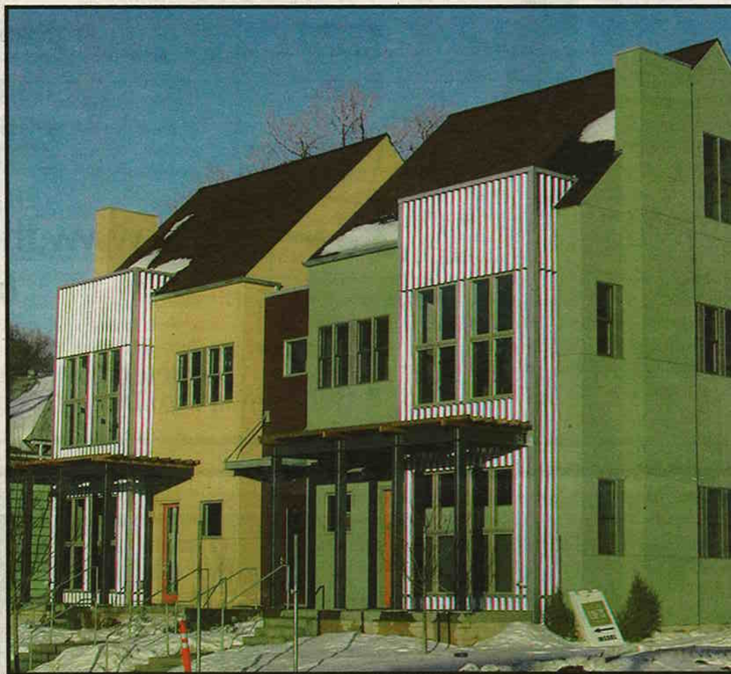
The three-story north building offers eight townhomes and eight one- or two-level flats.
