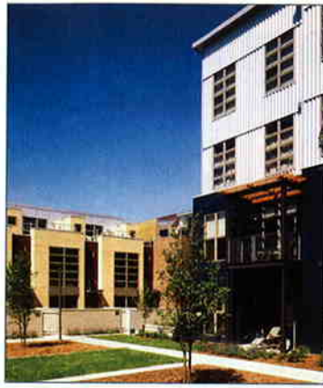
Midtown Exterior, Minneapolis, Minn.
